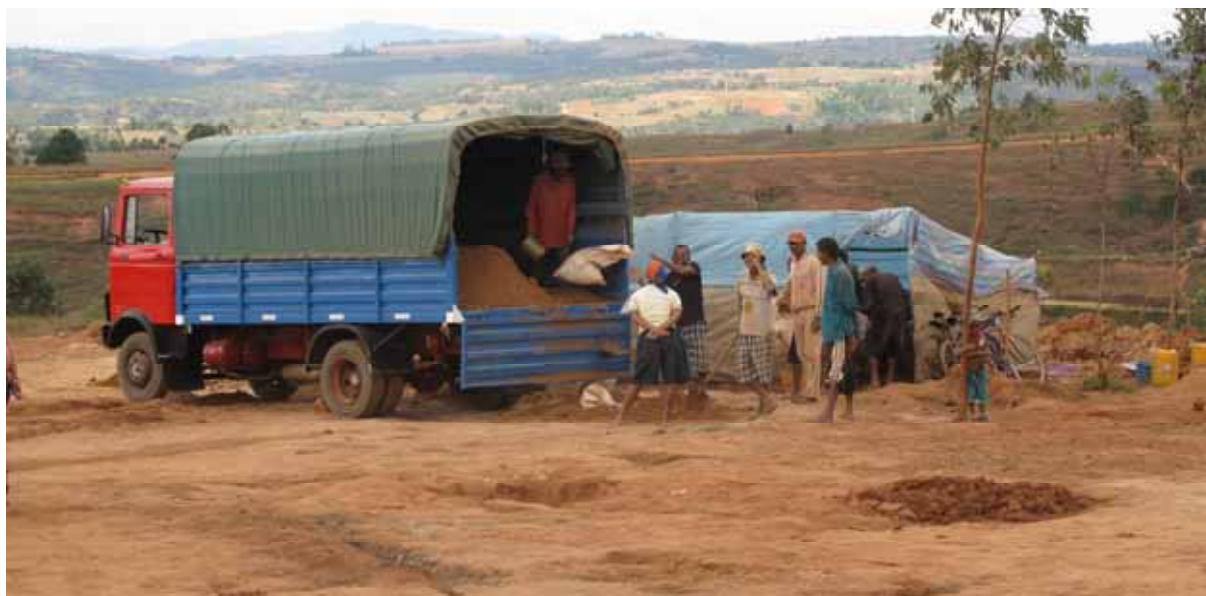
Figure 25: Lorry for transport of earth to river, Soamahamanina, near Arivonimamo
