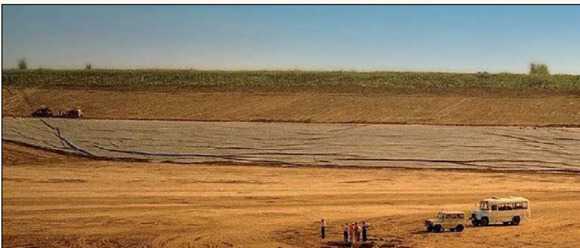
Figure 10: Black plastic liners installed at one mine site
