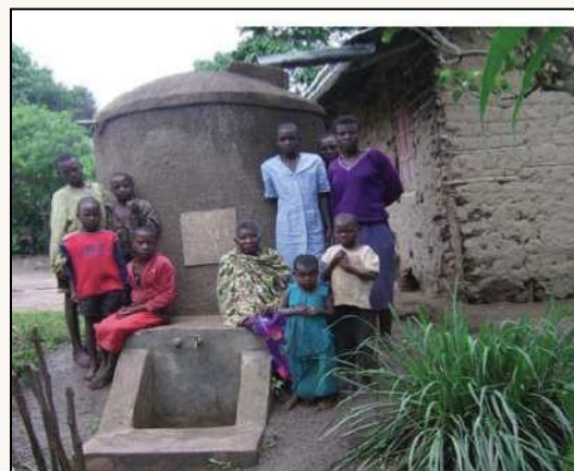
Figure 16: Rainwater falls onto this iron sheet rooftop and is diverted into a large tank.
