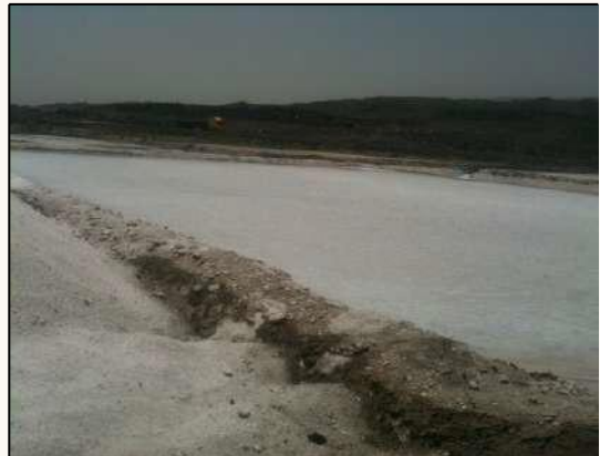
Figure 8: Sides of the pan are typically made up of the soil dug from the pan bottom
