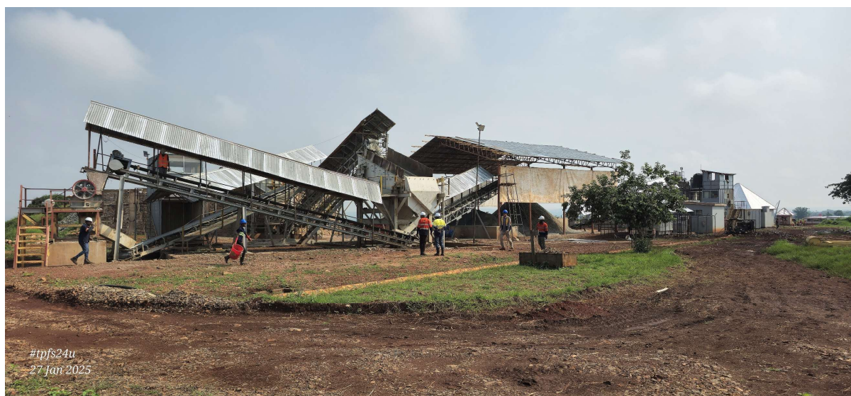
Figure 5: Crushing Circuit - Mwamba Processing Plant, Tanzania ©Mwamba
