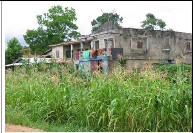
Plate 6.6 bombed out building in Koidu
